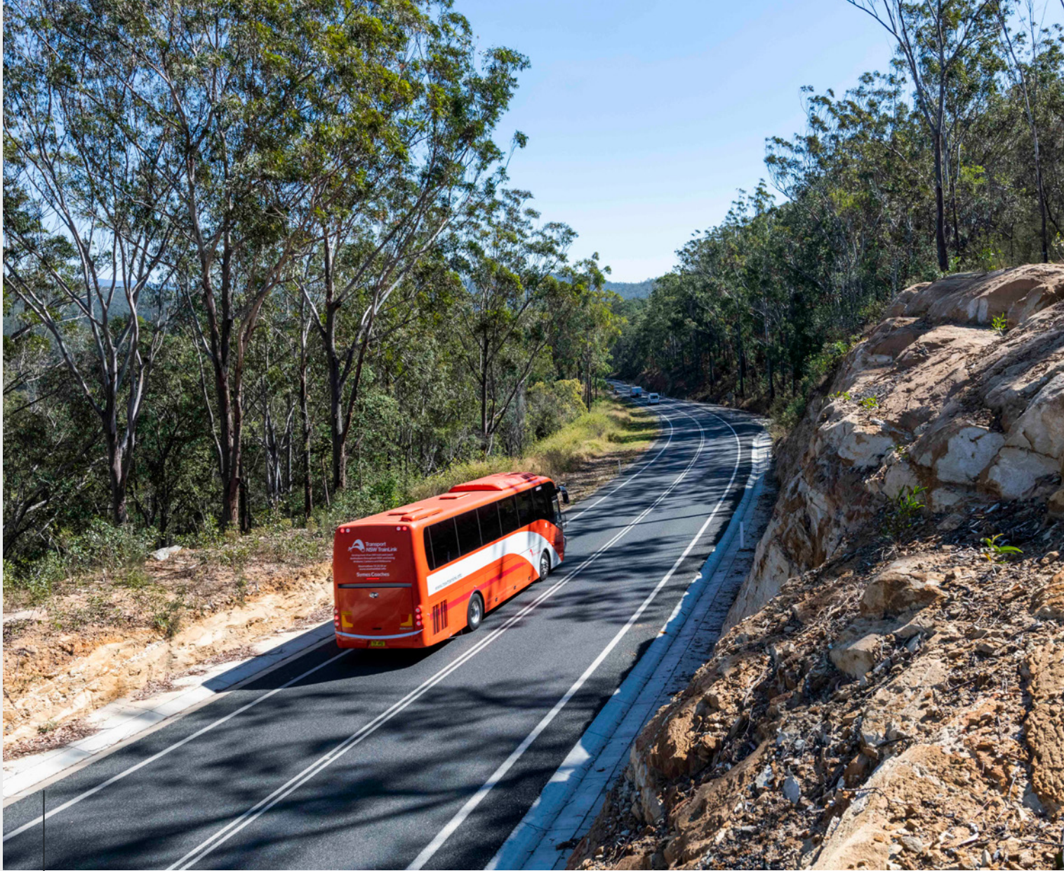
A newly repaired section of road built back to a more resilient standard following a landslide.
