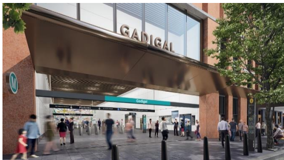
Sydney Metro names Gadigal Railway Station in Pitt Street, Sydney.
